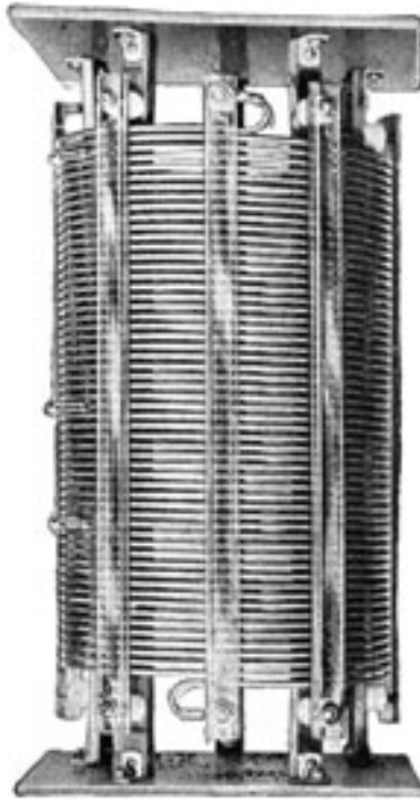
Figure 86.-Transformer used with transmitters.
